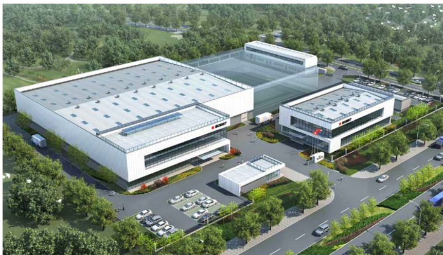
Aerial view of the new site project
