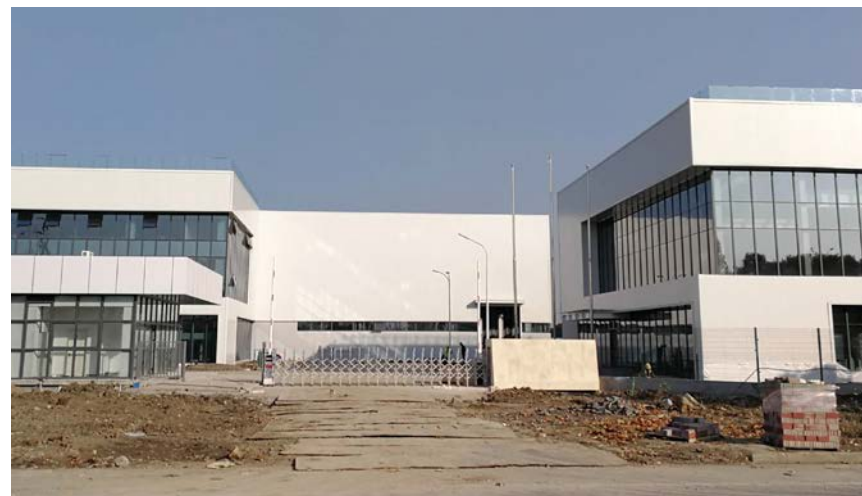
Front view of the new site project
