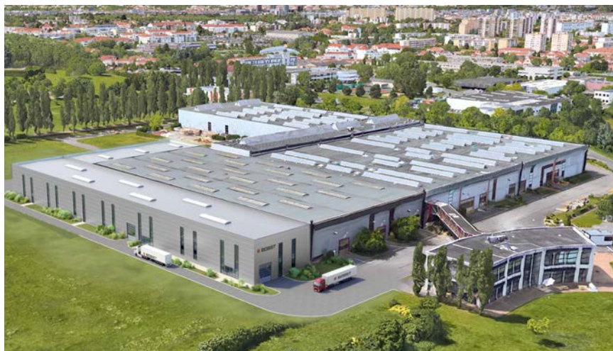
Aerial view of the new competence center
