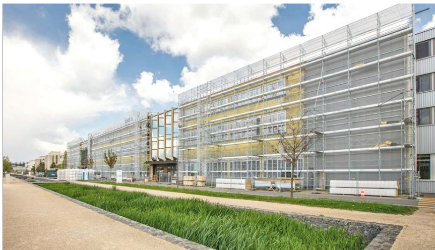
Facades renovation and insulation
